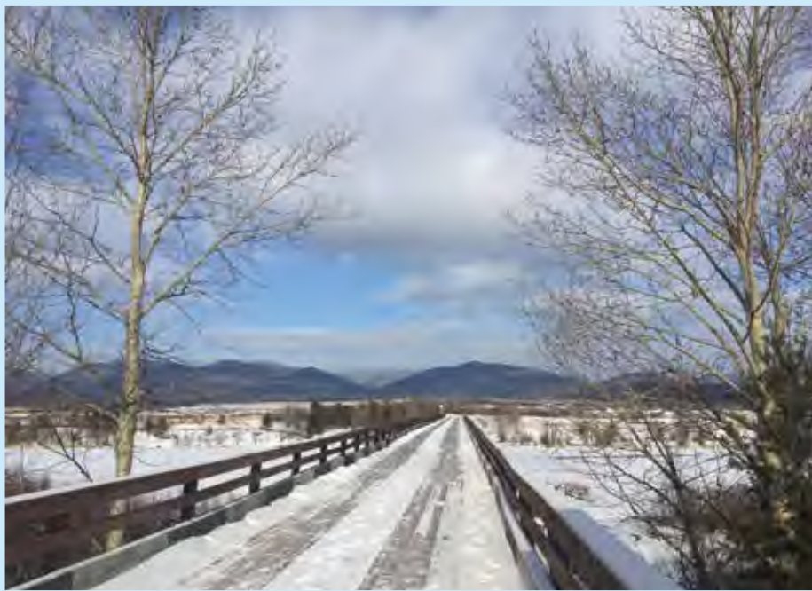
The Sungacha River Bridge after maintenance
