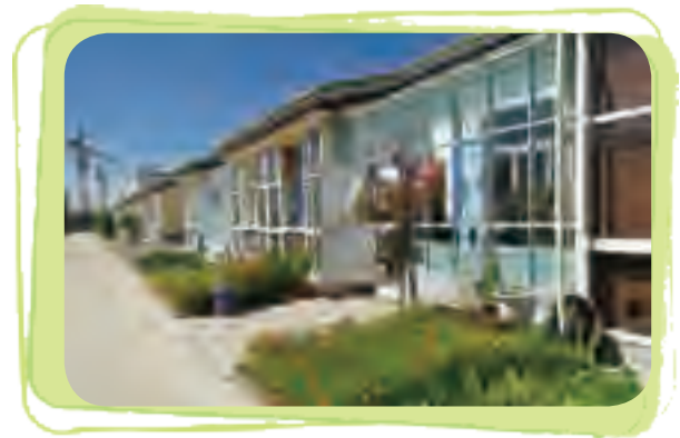
Settlement of Herdsmen Built by Shenhua in Shaliuhe town, Gangcha County of Qinghai
