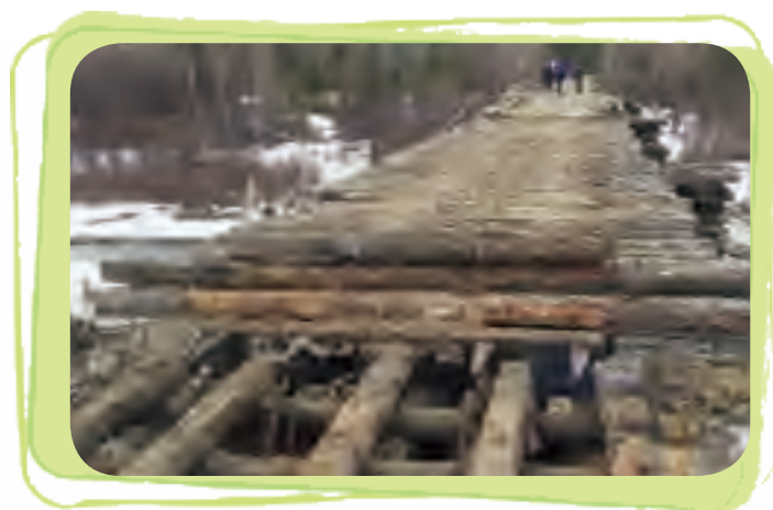
A Bridge is being Repaired Locally by Shenhua Russia
