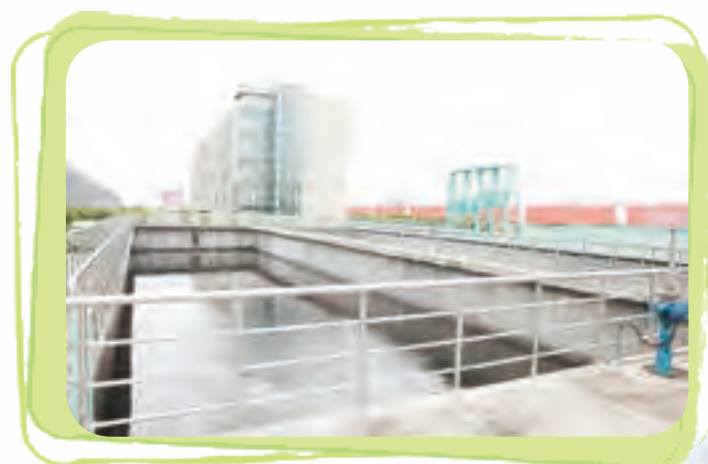
Collection Pool for Sewage
