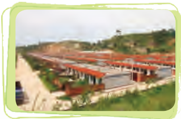
The Construction of a New Village Participated by Shenhua
