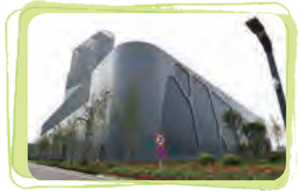
Digital Power Plant – Shenhua Guohua (Beijing) Gas Thermal Power Co., Ltd.
